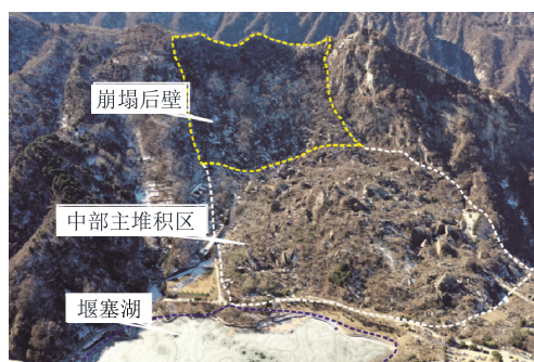
图1 水湫池崩塌体 Fig.1 Shuiqiuchi rock slope failure
